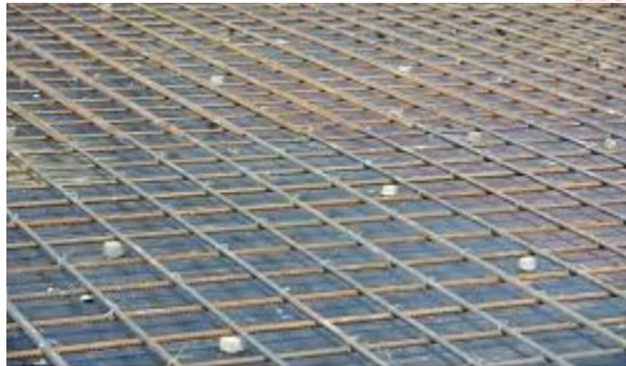
Concrete Cover Block in Slab
