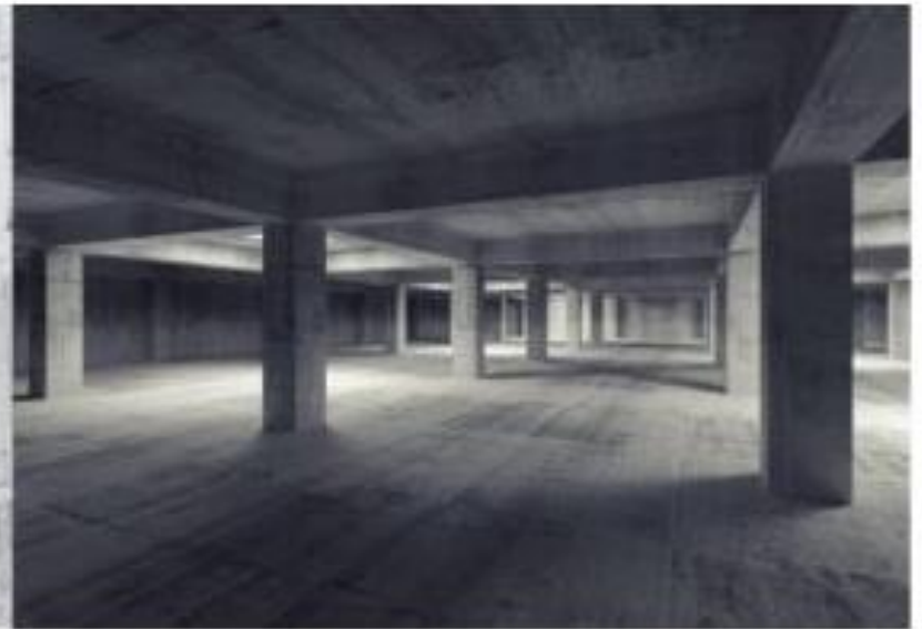
Conventional Slab- Beam System
