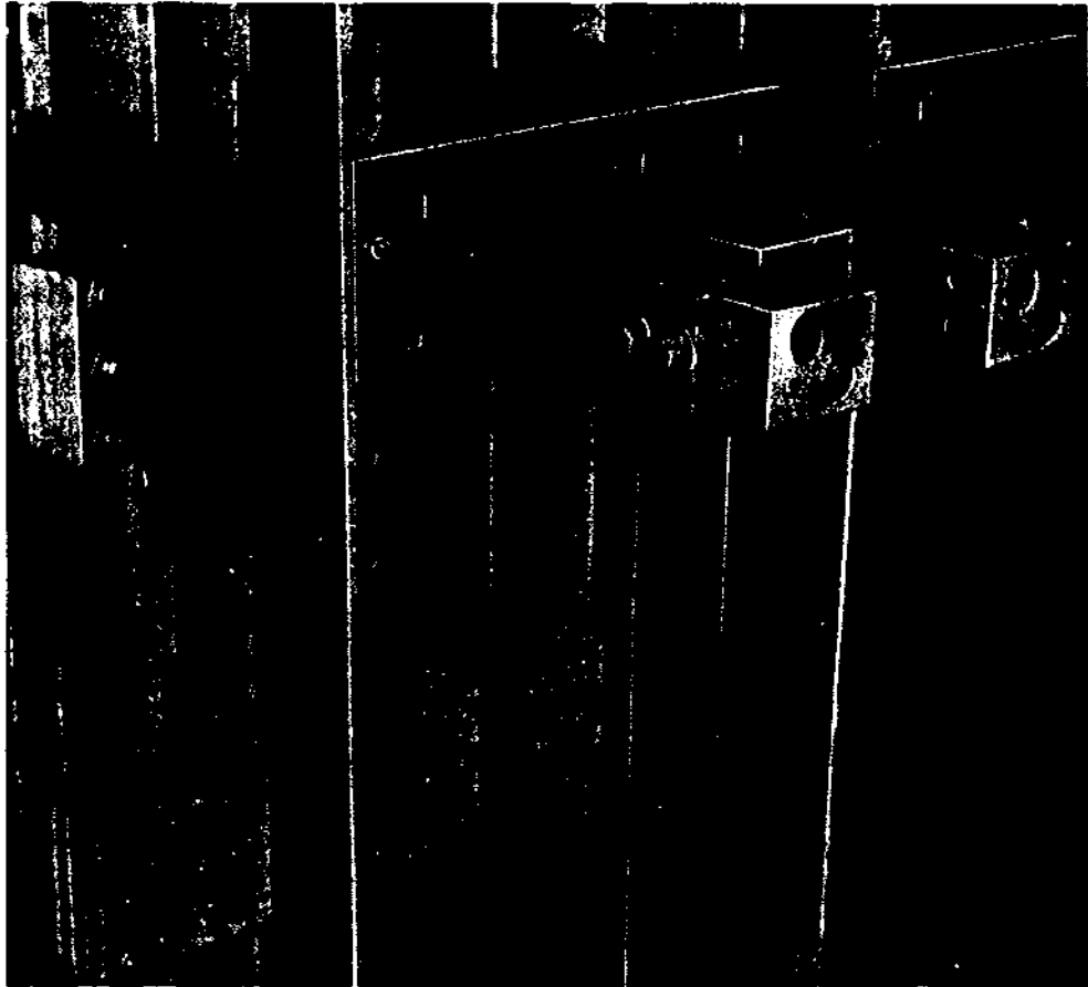
Fig. 16 – Rear Extensions Extend into the Cable Compartment for Termination of Feeder Cables
