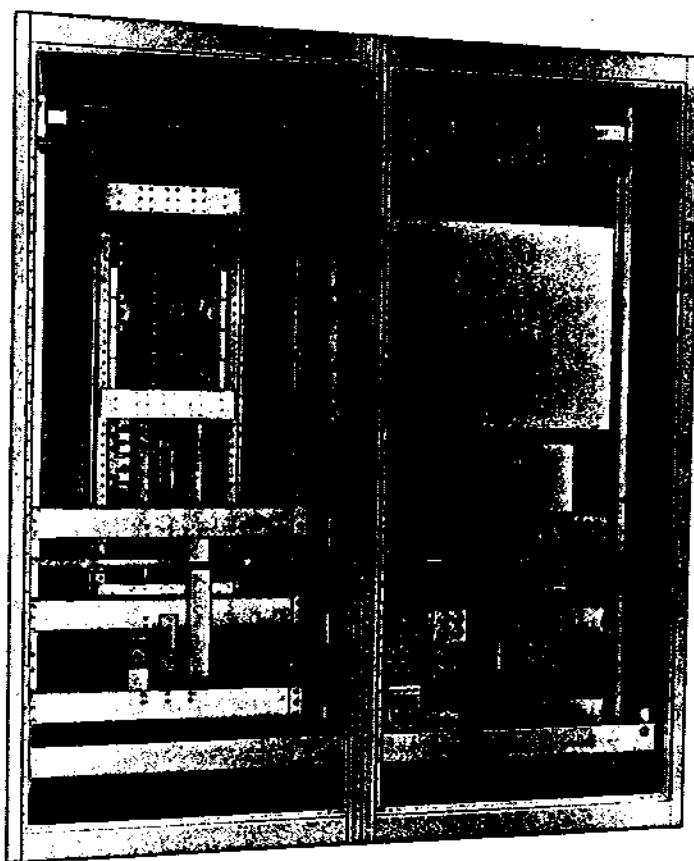
Fig. 9 – Front and Rear Accessible Switchboard with Panelboard Type Branch Circuit Devices
